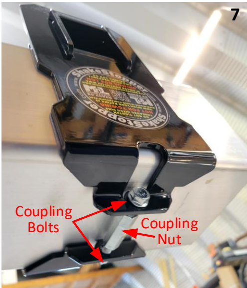
7. Connect Face Plates using Coupling Nut and Bolts. Finger tighten only. Seeing exposed bolt threads is okay.
